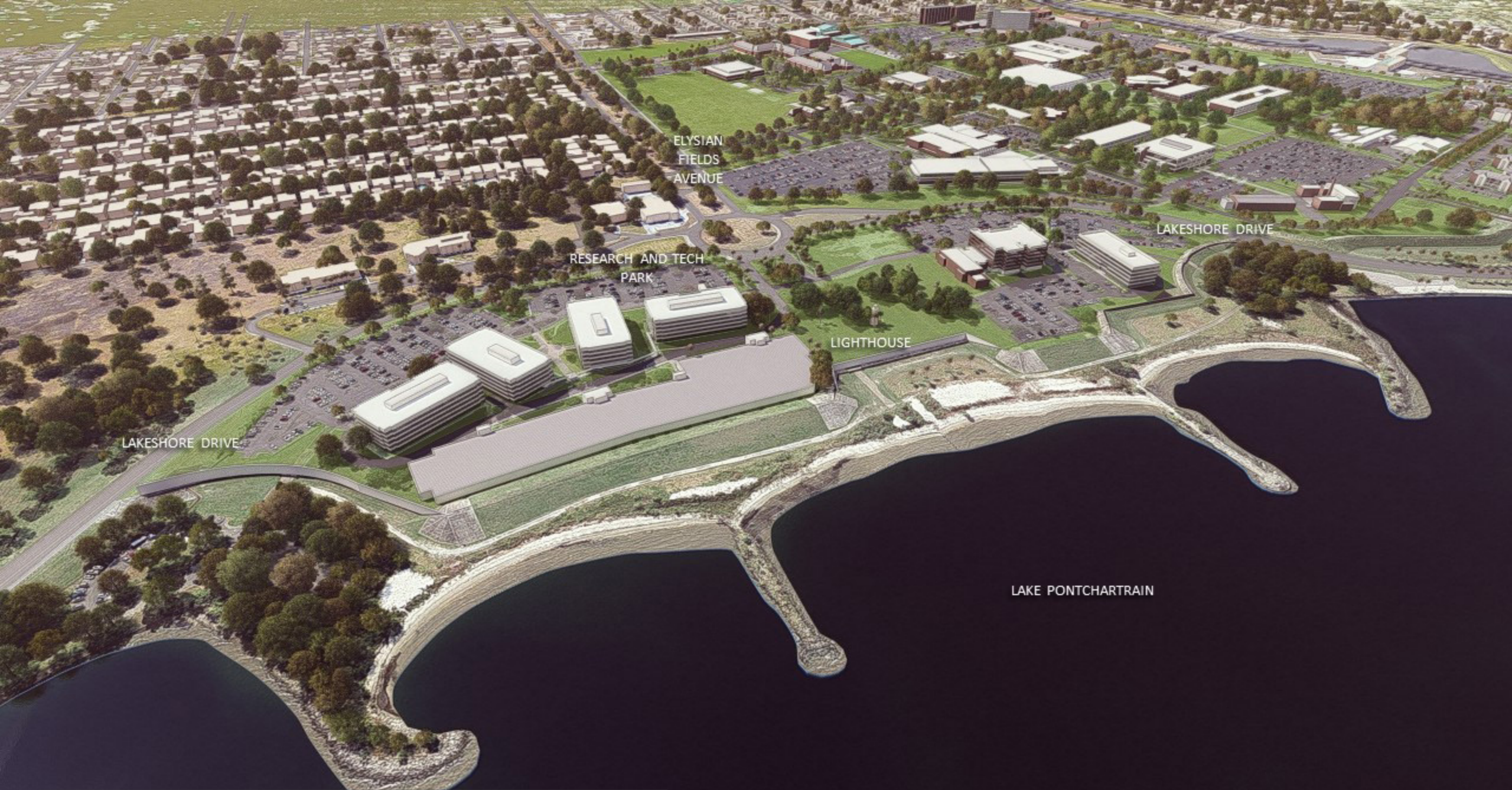
VIEW OF RESEARCH AND TECH PARK FROM NORTH - EXISTING CONDITIONS
