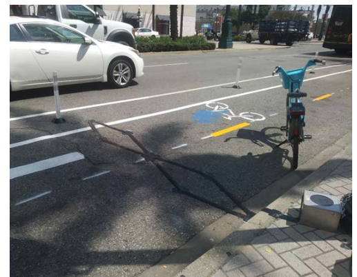
Figure 2 EcoCounter EZ-Zelt temporary inductive loop counter, installed on temporary protected cycletrack, Canal Street, New Orleans Photo Credit: Tara Tolford
