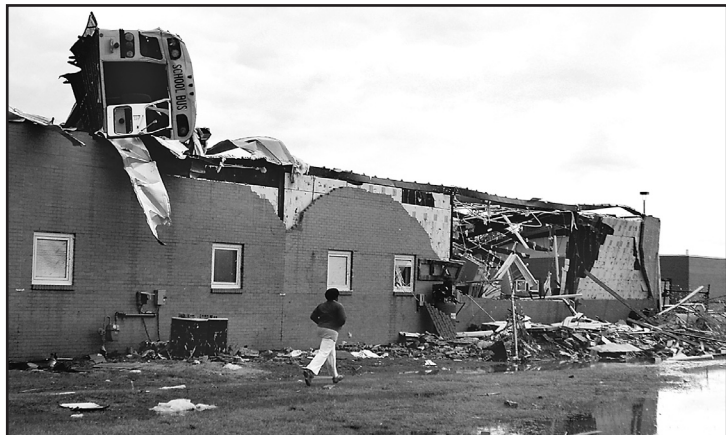
Figure 7-2. A school bus was lifted atop a section of Caledonia High School, Caledonia, Mississippi (January 2008)
