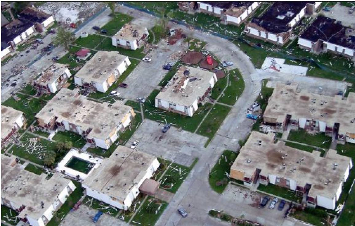
Figure 7-46 Wind Damage from Hurricane Katrina – Estimated Wind Speed 105 mph)
