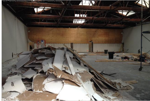
Wet dry wall is removed from an art gallery in the Chelsea neighborhood of New York following Hurricane Sandy. Photographer: Katya Kazakina/Bloomberg
